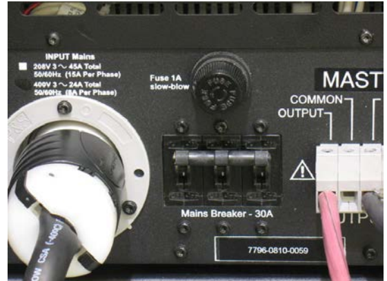
Figure 3.2 4301-60 Back-Panel Power Switch/Circuit Breaker
