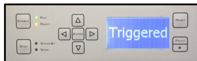
Figure 4.4 Test Successfully Completed
